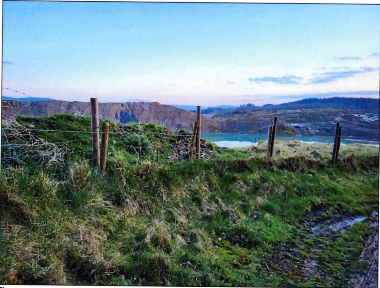
Figure 5: Inadequate fencing around the silt pond.
