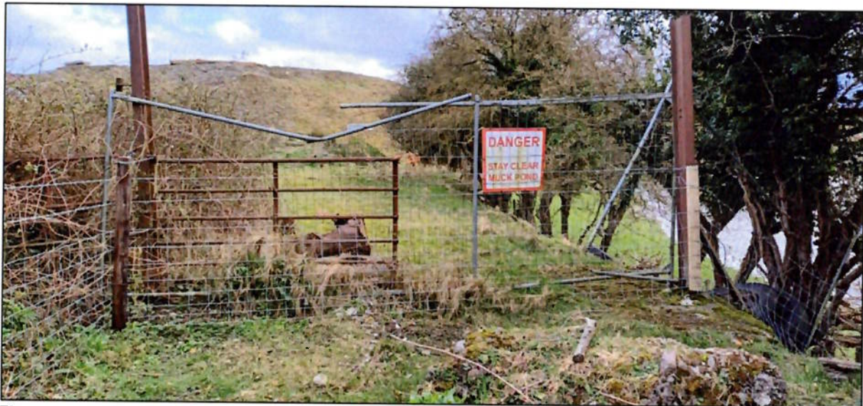
Figure 2: Lack of adequate fencing as required under Condition No. 20 of Reg. Ref. 07/267.
